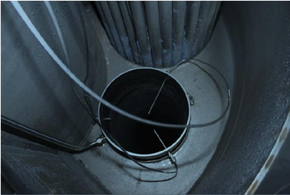
Figure 10: Picture of the real separator zone of the CIRCE facility. The 91 double bayonet tubes of the HX are depicted, together with the riser outlet and its three thermocouples. [1.]
